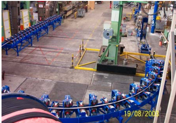
Photo 2: 180° loop between lead extruder (right) and outer sheath line (left)
